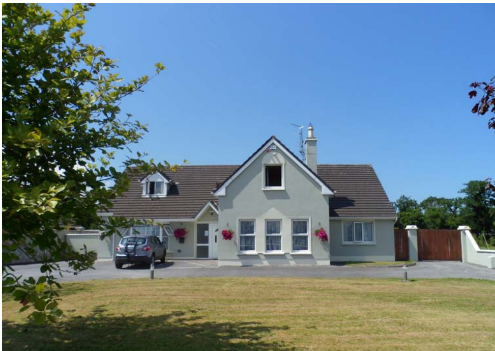
Knocklee House, Tralee, Co. Kerry
